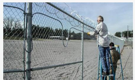
Integration with Fibre Optic Fence line
